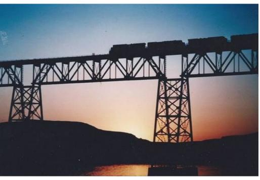
reported to be the last major "hot rivet" railroad bridge built in the west, although verification is elusive. The bridge was the centerpiece of a new direct and more efficient U.P. line reaching into the Inland Empire. The rail is 240' above the water. The bridge crosses the Snake near Starbuck, Washington, once an important UPRR town.
